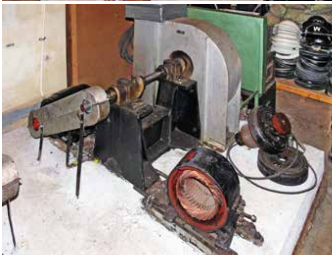
Interior of the plant room. Photo Victor Smith
